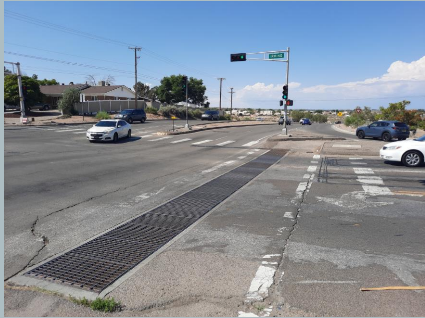
View north from SE corner
